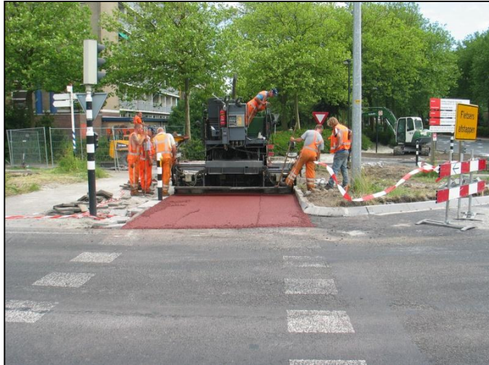
Figure Paving colored asphalt
