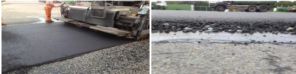
Figures 7 and 8: Applying the binder course preparation section and cross-section of thin binder course
