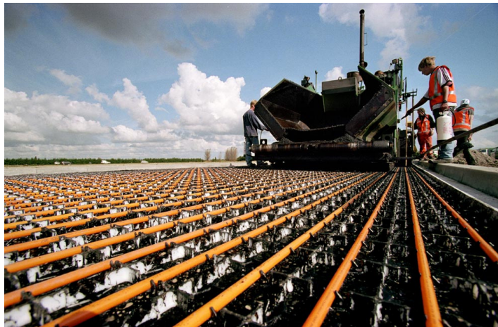
Figure 4. Overview of Final Asphalt Solar Collector System
