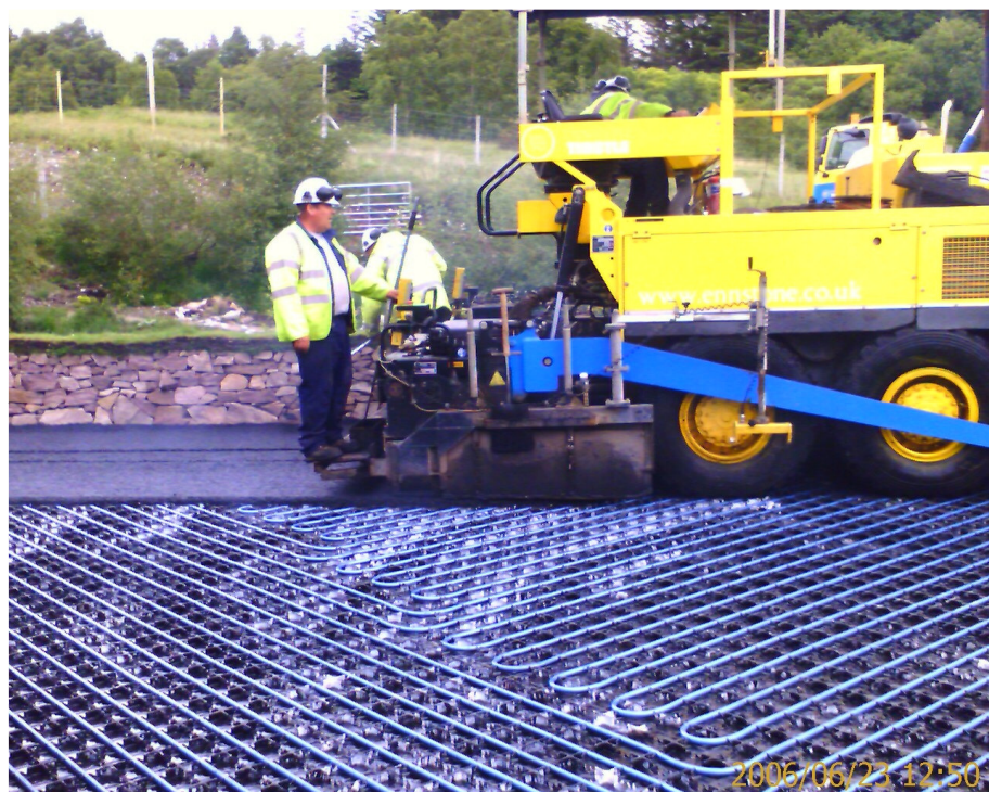
Figure 9 Asphalt Solar collector under construction in Ullapool Scotland June 2006.
