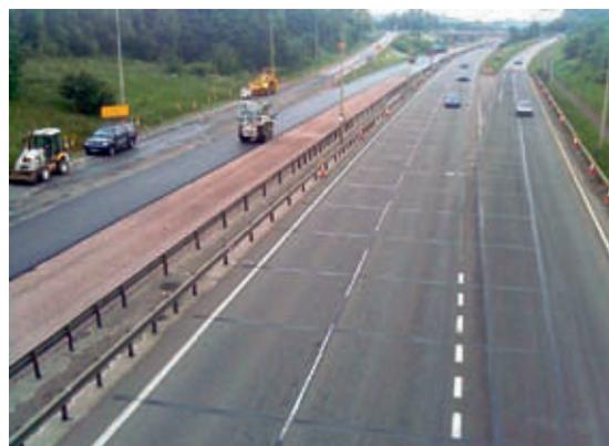
Picture 2 – Highway prior to treatment (right side) and during overlay (left side)
