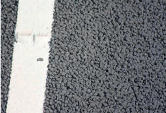
Picture 4 – Final texture at >97% compaction.
