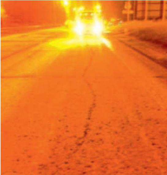
Picture 3 – Longitudinal cracks revealed after night time removal of Safepave® and 20mm of concrete surface.
